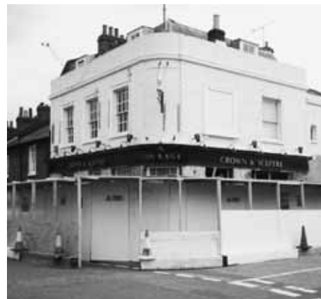
. . . and after stripping the tiles
