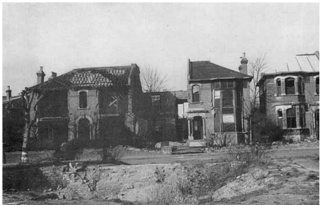
Breakspears Road: damaged house, front exterior
